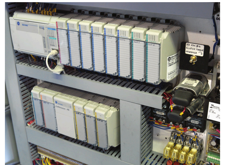
A series of Allen-Bradley Micro-Logix PLCs (programmable logic controllers) forms the heart of the SM3600 labeler's control system.
